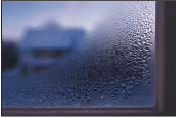
Condensation on the inside of a windowpane.
